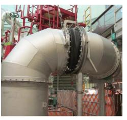
Quick Disconnect Ductwork Connection
