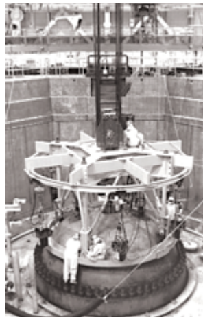
U.S. plant outage showing six TENSOR tensioners, a rigid pole system and head lift rig/carousel
