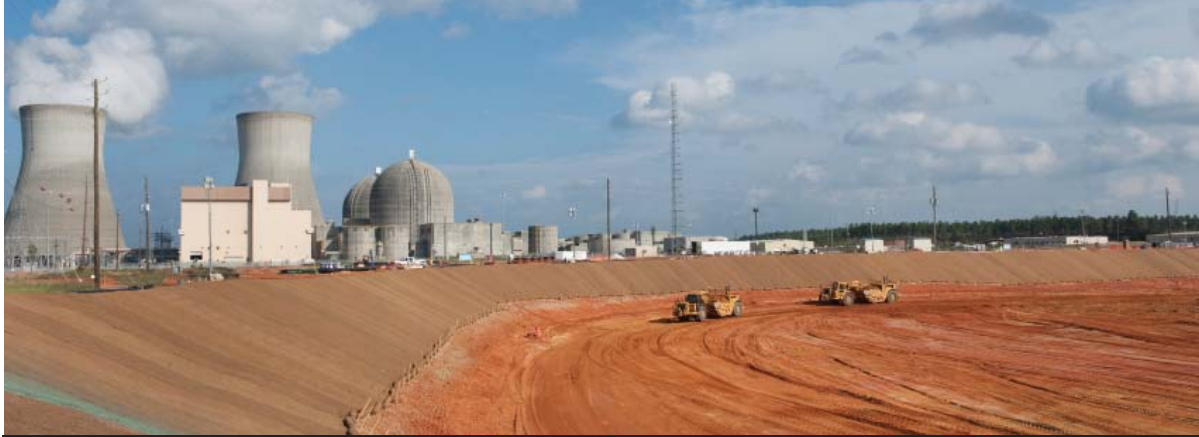
Plant Vogtle Construction/Units 3 & 4/October 7, 2009
