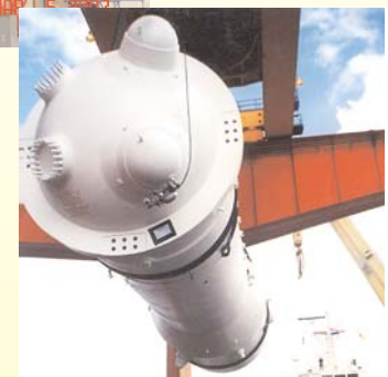
Replacement Steam Generator at Comanche Peak
