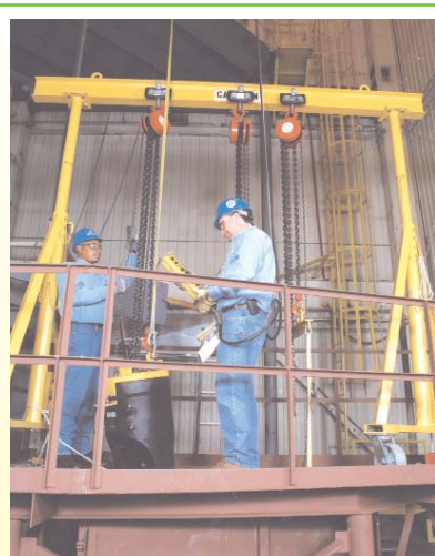
Rigging mockup for typical Mechanical Stress Improvement Process reactor vessel nozzle sandbox configuration.
