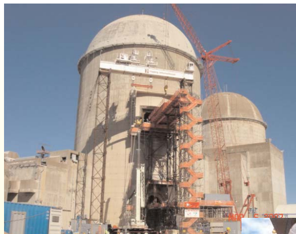
Replacement Steam Generator at Comanche Peak
