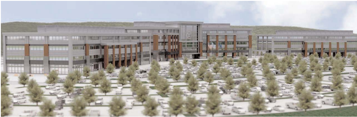
The Westinghouse campus north of Pittsburgh, Pennsylvania, United States will offer ready access to the Pittsburgh International Airport.
