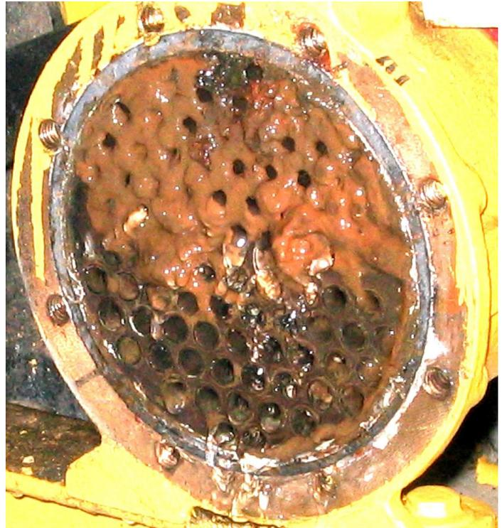
Condensate booster pump heat exchanger before cleaning
