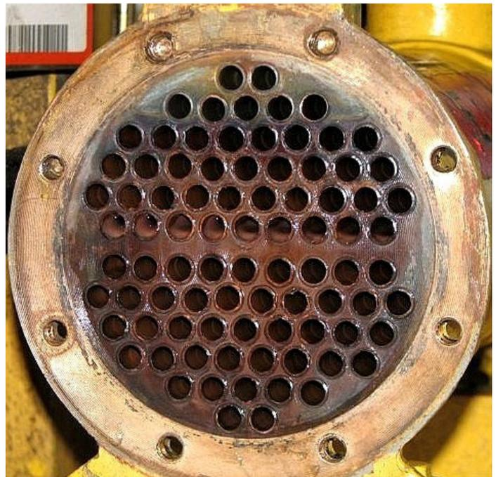
Condensate booster pump heat exchanger after cleaning
