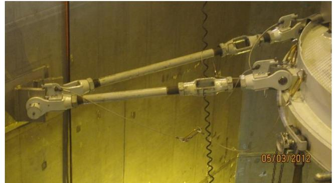
*CRDM Seismic Support*
