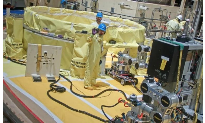
Installing Gemini robot through RVH stand manway.
