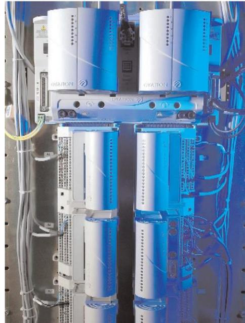
*Redundant Controller and Local Input/Output Modules*
