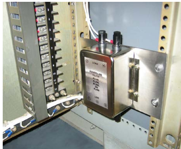
Power Line Filter Installed in Rear of NIS Console Bay
