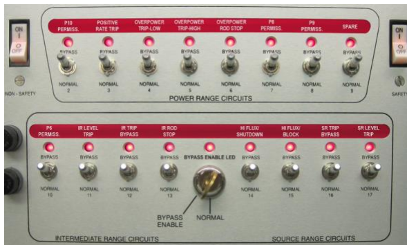
Source, intermediate and power range bistable signals can be bypassed for no-risk testing and maintenance.
