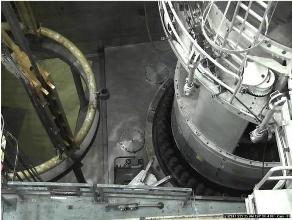
View of Narrow Gap Permanent Cavity Seal Ring Prior to Cavity Flooding with Hatches Installed
