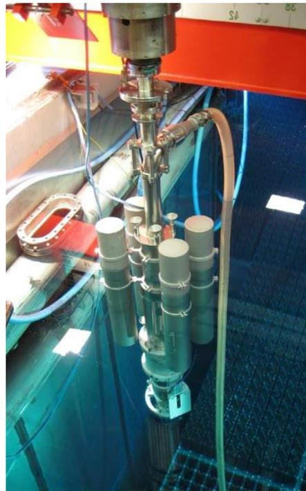
*Operation of FAST Equipment in a German Nuclear Power Plant – including 4 floating tanks for weight reduction*
