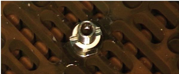
Completed instrument tube tie rod installation
