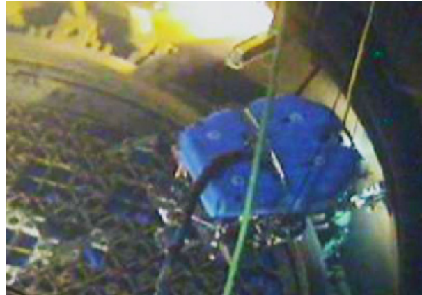
JAIMS performing jet pump diffuser and adapter weld exams
