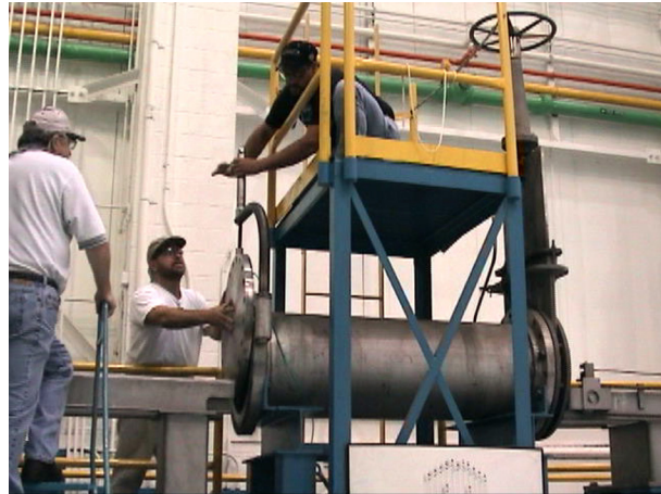
Personnel working on the fuel transfer tube
