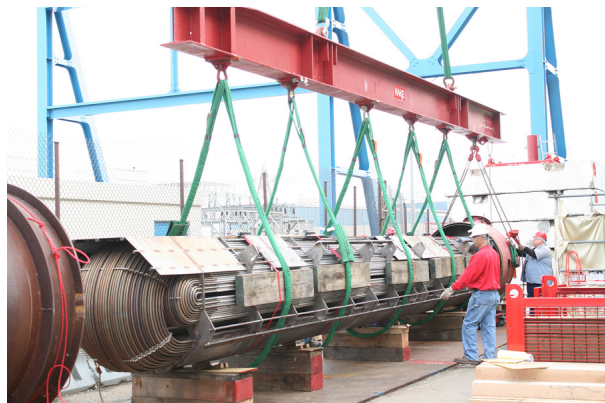
Workers replace feedwater heater bundles
